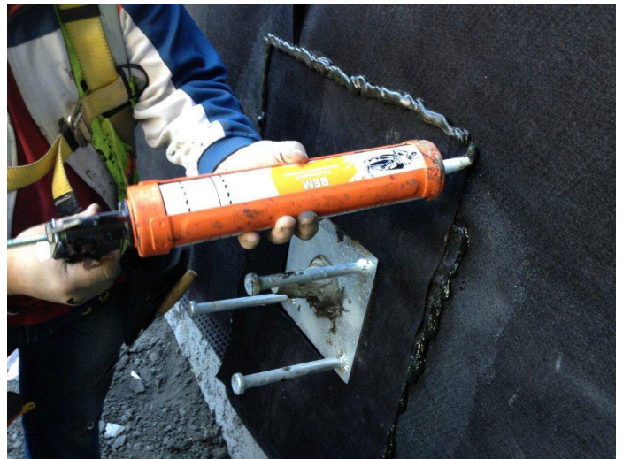
Installer for CHM Weatherguard details a Nelson Stud PRECON® tieback using BEM, a one-component, ready-anytime membrane. The PRECON system with BEM helped reduce detailing time on the D/FW rail station project by 35%-40%.
