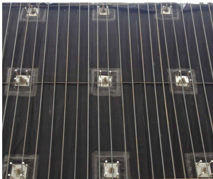
Running rebar over finished, fully detailed PRECON installation, prior to pouring concrete. The concrete "grabs" soil nails protruding from Nelson Studs, strengthening the structure and, as concrete cures, PRECON forms a mechanical bond for a secure, waterproof installation.
