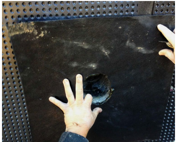
PRECON flap over MEL-DRAIN being fitted around Nelson Stud center/soil nail screw before the base plate and anchor bolts are installed.
